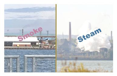
While not harmless, the steam cloud coming out of the quench tower is far less destructive than what comes out of the main stack, which is not always as visible.
